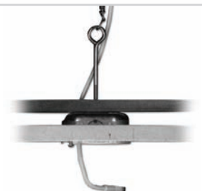
Occupancy Sensor Installed with J-box Installation Time: 45 minutes
